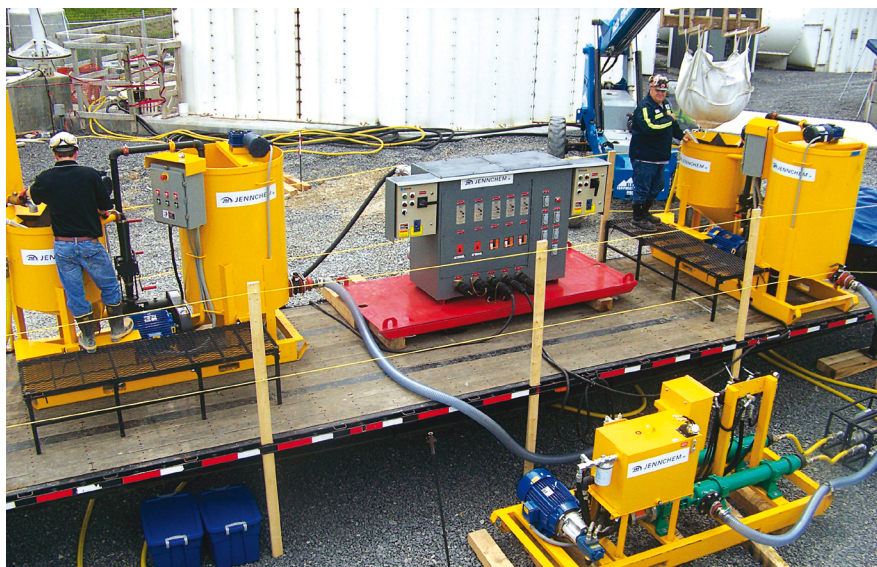
Trailer mounted, electric powered operations.
